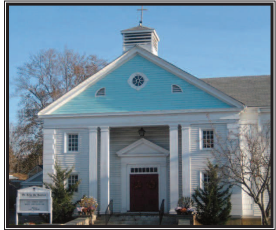
St. John the Baptist Church 52 Main St. Essex, MA 01929-1343 Established 1931
